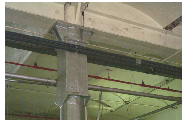
View of interior structure
