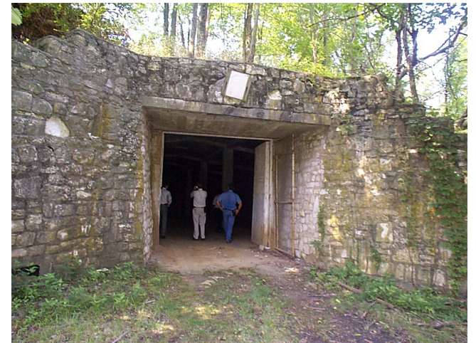
Existing view of North elevation
