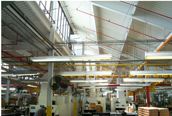
Existing Interior View
