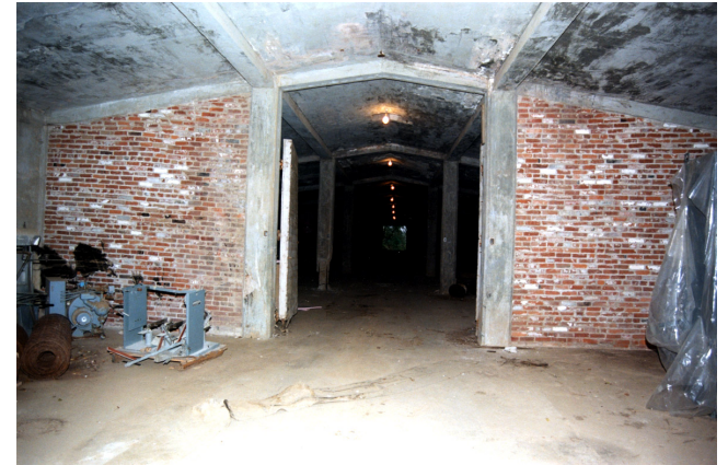
Existing view of interior
