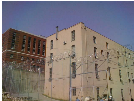
Northeast corner of building, H.U. 5 is in the background
