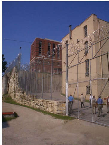
Existing view of Northern end of pre-1885 wall @ Shoe Factory
