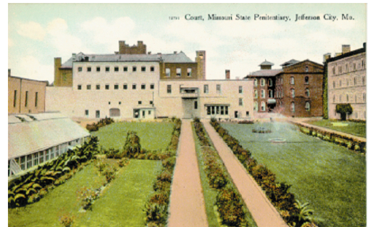
Historic View of East Elevation prior to WPA (1936) additions, the rear pre-1885 structure is shown here.
