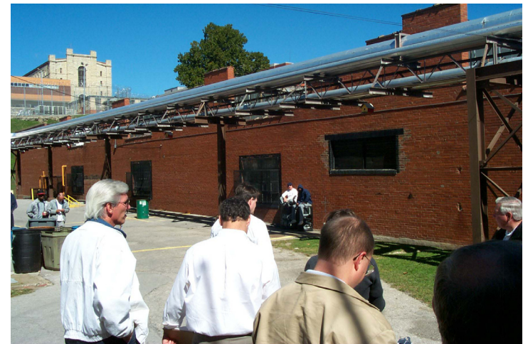
Existing South Elevation, above grade steam pipes are in the foreground
